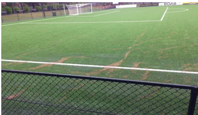
Photo 24: Organic infill displaced after rain, needs to be brushed to redistribute infill by using specialist machinery that can collect it and redistribute it accordingly. (Source: Smart Connection Consultancy)
