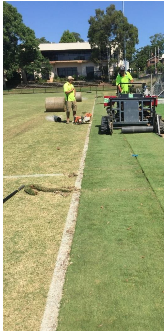
Photo 17: Lines person running lines being reinforced with hybrid technology (Source: HG Sports Turf)
