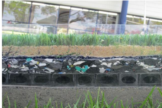
Photo 14: Example of horizontal drainage cell under shockpad (Source: Wayne Stuart - City of Swan, WA)
