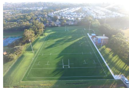
Photo 2: Rugby Union - Latham Park - NSW (Polytan installation)
