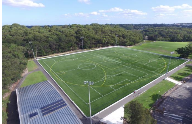
Photo 29: Blackman park, Lane Cove NSW - Installed by Team Sports (Source - Lane Cove Council)
