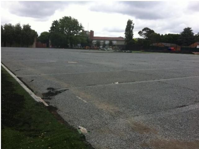
Photo 5 Ag drains to have a tendency to move after installation which impacts on the surface
