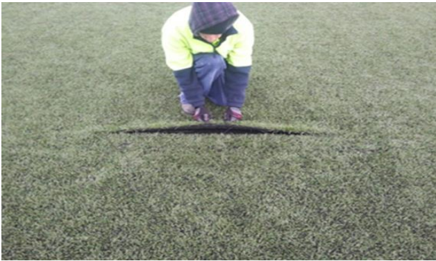
Photo 10: Example of seam failure
