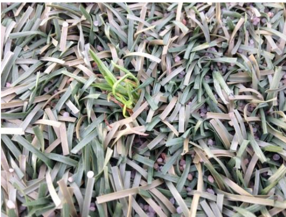
Photo 22: Turf not maintained adequately is showing the yarn is being bent over due to lack of adequate infill and weeds are being allowed to grow
